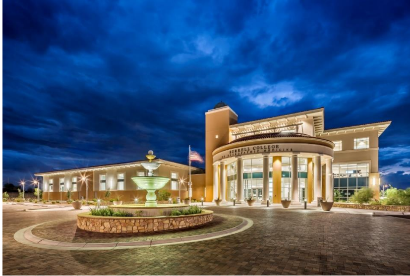
Picture depicted is of the New Mexico Campus
